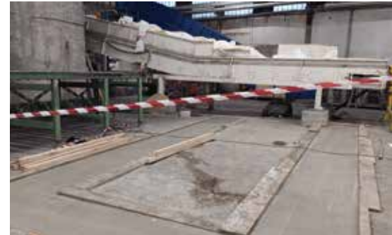
Foundation built for the guillotine.
